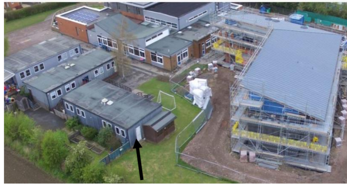
Year 3 and after school club were in these porta cabins.
